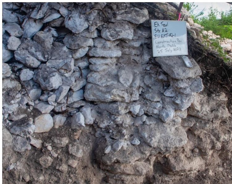
Figure 16: Photograph of construction pen (stacked stones in center of photo) in north baulk.
