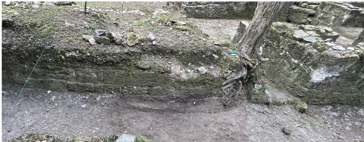
Figure 4: Modified bedrock drain exposed in Unit CTB3W-2022-2, along the southern wall of Structure B9.
